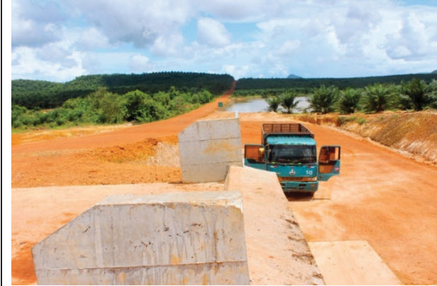
At Estate B: New loading ramp facility
